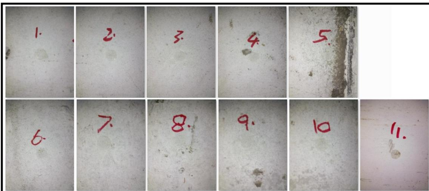
Figure 7: Surface damage by small hard body impact - closed up view of indentations
